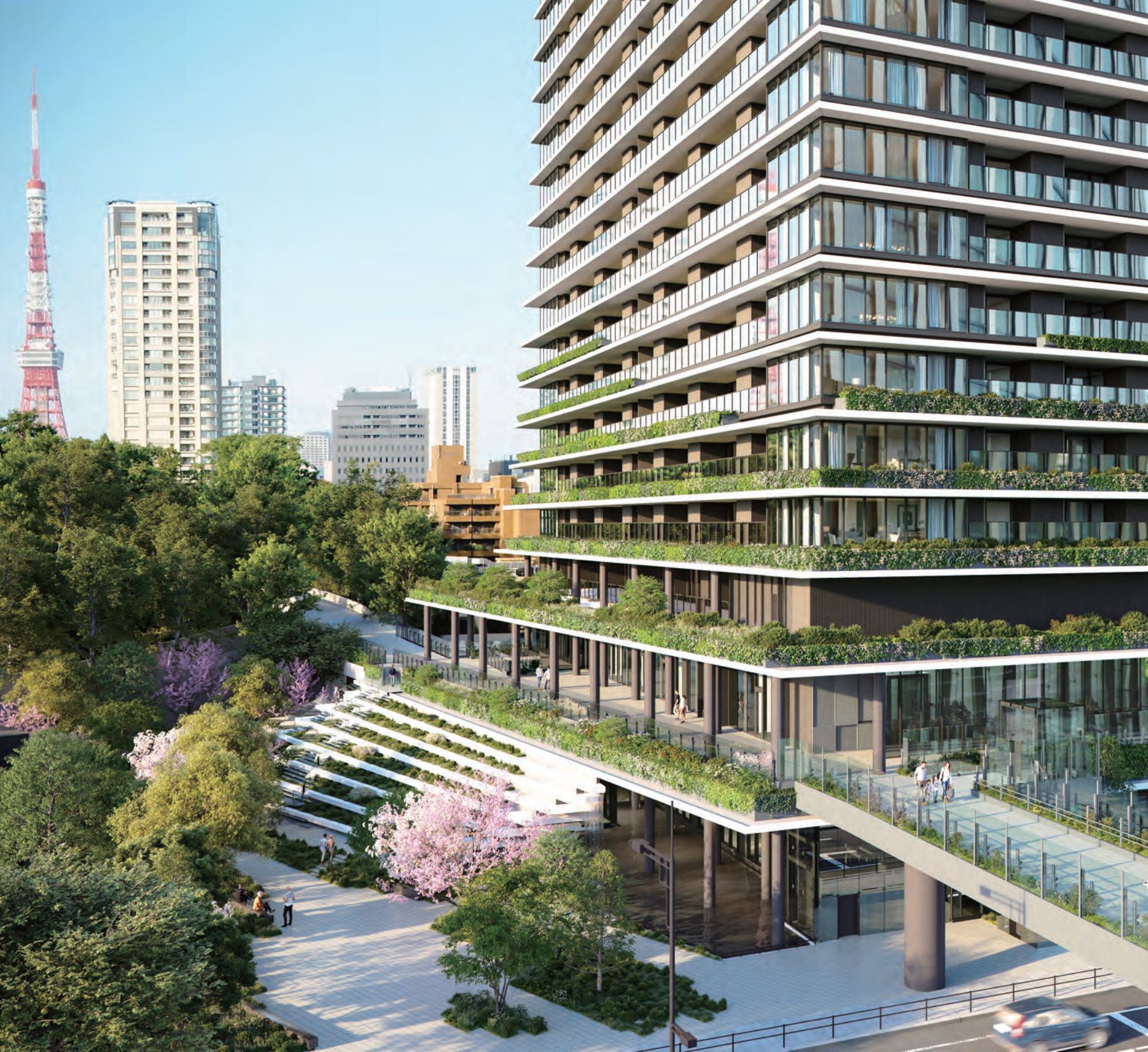
Toranomon Hills Residential Tower | 外観
